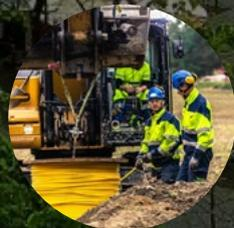
Trenching by Elenia during installation of underground services conduits to replace overhead wires.
